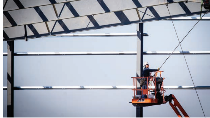
The steel skeleton of the Hughes Fieldhouse began rising from the ground this fall.
